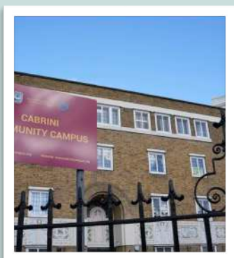
Entrada do Cabrini Community Campus
