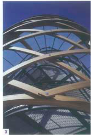
1. 3. Uffici Hugo Boss Industries Switzerland offices in Coldereris 2. 4. Tortona 37
