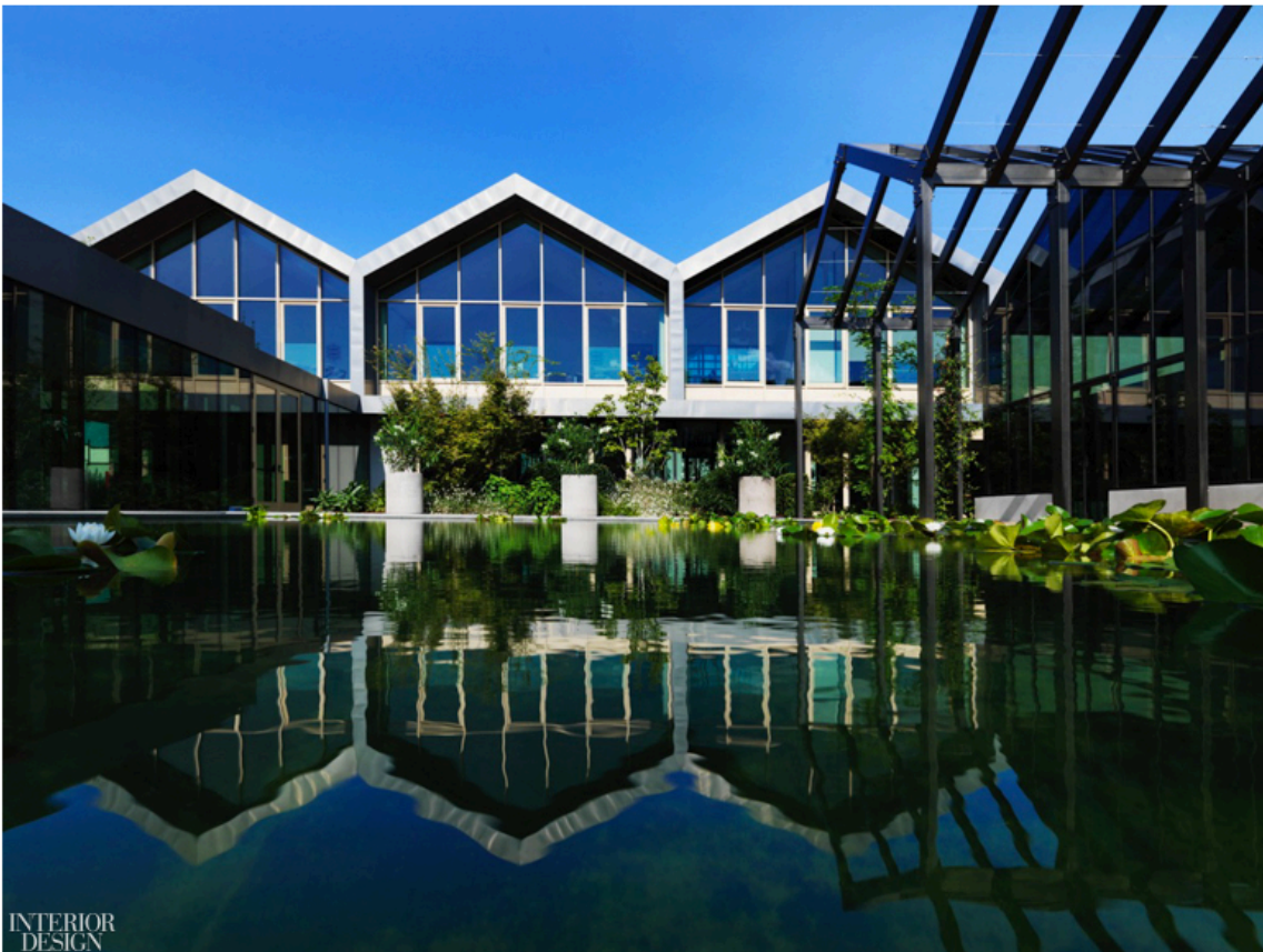
The Davines headquarters in Parma, Italy by Matteo Thun & Partners. Photography by Andrea Garuti, courtesy of Matteo Thun & Partners.
