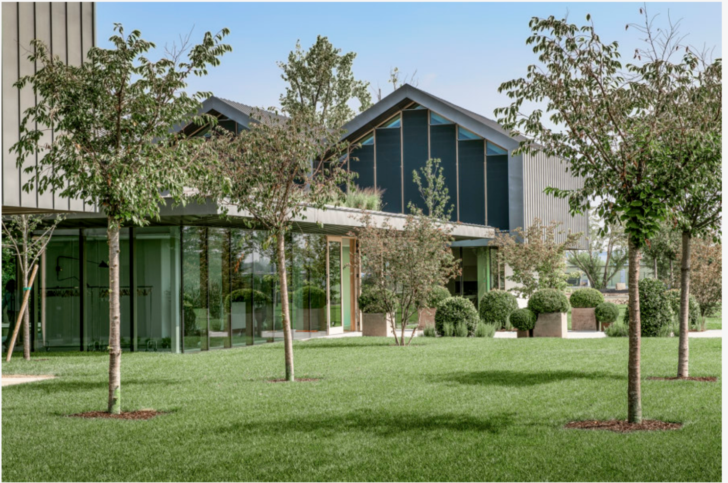
The Davines Village project used certified suppliers and materials such as innovative cement and active anti-pollution components. Photos: Max Zambelli (top, middle), Andrea Garret (bottom)
