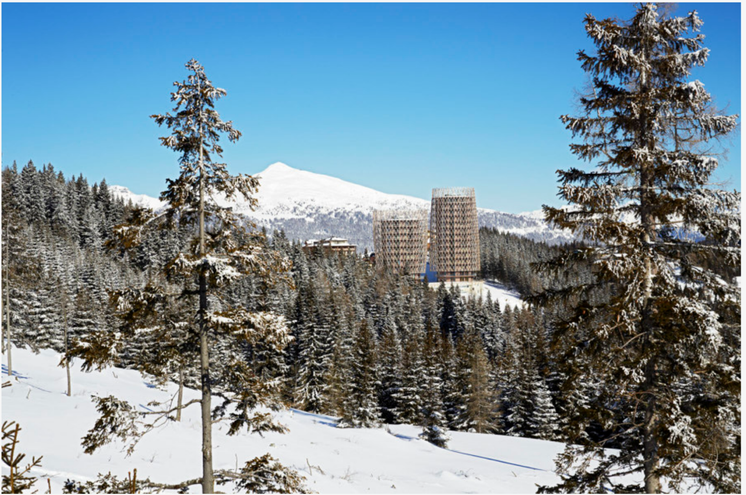
Matteo Thun & Partners' Mountain Residence Towers are vertical landmarks clad in larchwood, connected with a biomass generator. Photos: Jens Weber
