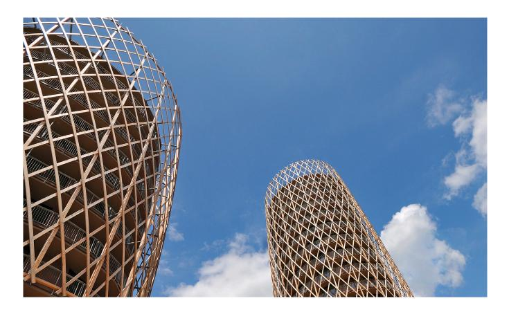
By following the motto 'kilometre 0', wood, the main building material, once again stands up to the test. The two cylindrical structures are wrapped by a round bodied diamond rhombus structure made from local larch wood that symbolizes the direct association to the environment, fusing the inside and the exterior.
